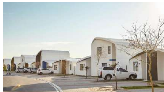
Completed units at Central Blue. Source: Citra
