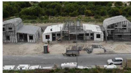
Houses under construction at Central Blue. Source: Citra
