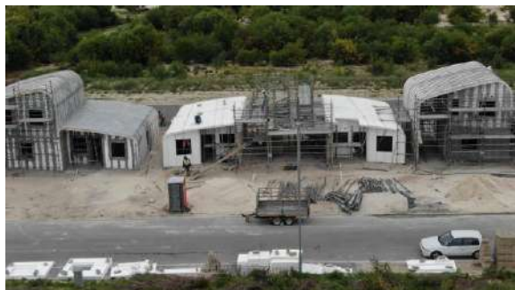
Houses under construction at Central Blue. Source: https://www.auhf.co.za/auhf-conference-2022-a-green-urban-future-for-affordable-housing/ .
