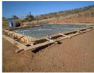
Raft Foundation as per Engineers Specification 25MPa - 20th of October 2012
