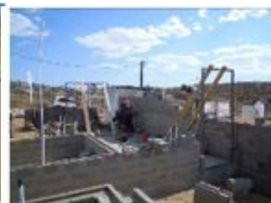
140 Thick Wall Super structure 27th of October 2012
