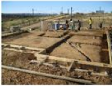
Form work for floated foundation 18th of October 2012
