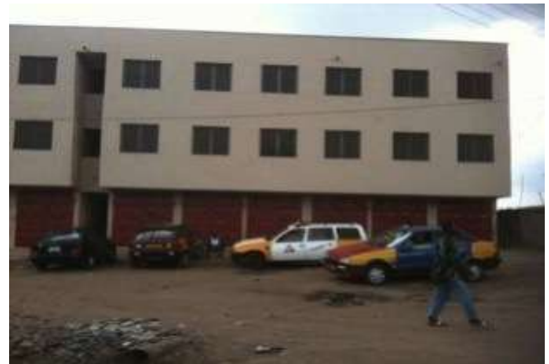
...replaced by 31 unit mixed-use, mixed-income building
