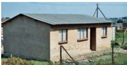
Houses built by AUHF member, Mpumalanga Housing Finance Corporation. See page 3.
